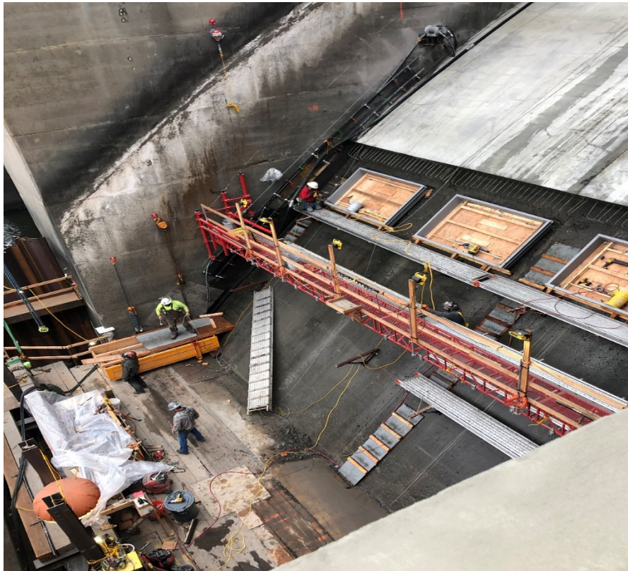
Figure 17. Antennas added to the Spillway at Lower Granite Dam
