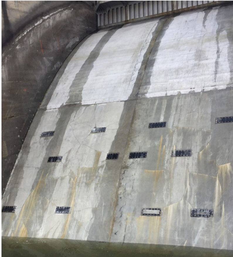
Figure 2. Lower Granit Dam Spillway interrogation site displaying the black covers that allow access to the antenna components for maintenance.
